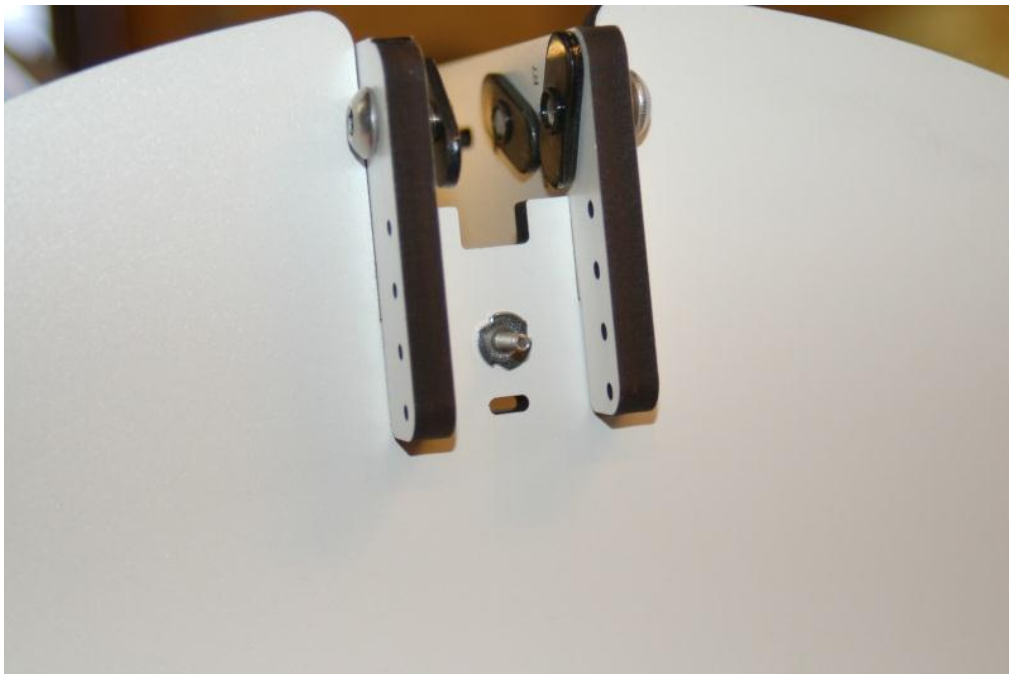
Figure 35 - Mounting Screw and T-Nut
